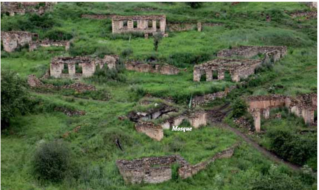
Photos 6. The remnants of the demolished mosque in Bashlibel (2023)
